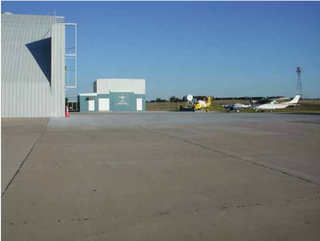
Gami Engine test building.
